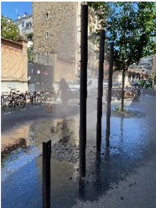
The street is closed to traffic and equipped with misting devices. When a button is pressed, a fine mist is released for a few seconds.
