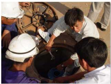
Water supply project at Phnom Penh
