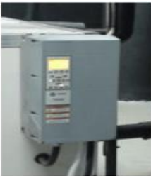
VARIABLE SPEED DRIVE
