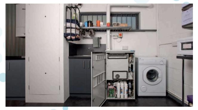
With the help of REBus expertise, the pilot has generated 3156 kWh in its first 85 days. Estimated net savings for the pilot will amount to 19.96% in Year 1, rising to 36.4% by Year 10. CO2 mitigation is estimated as 3 – 4 tonnes per
