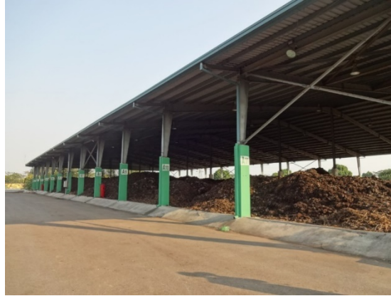
Large scale composting of municipal solid waste
