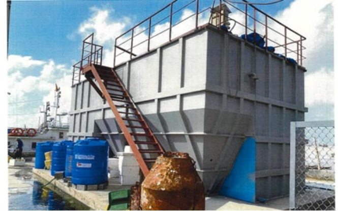
Sewage treatment facility
