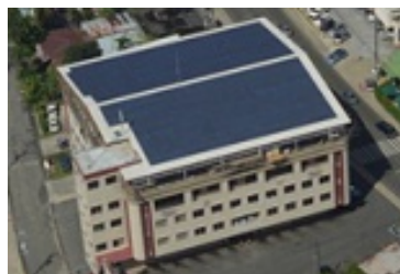
Installing solar PV system
