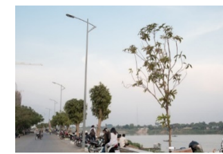
LED street lighting system
