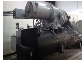
High efficiency air-conditioning and process cooling
