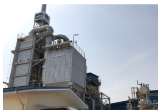
Waste to Energy Plant.
