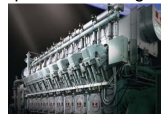
Co-generation system at factory
