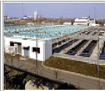
Waste water treatment
